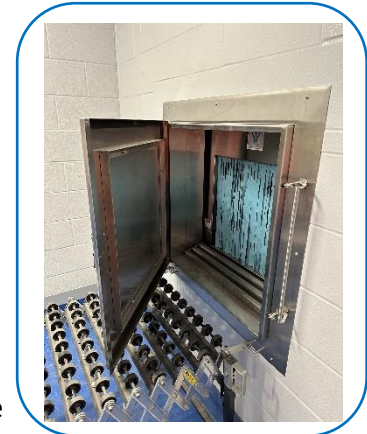
Pass-through Door & Off-load Conveyor
